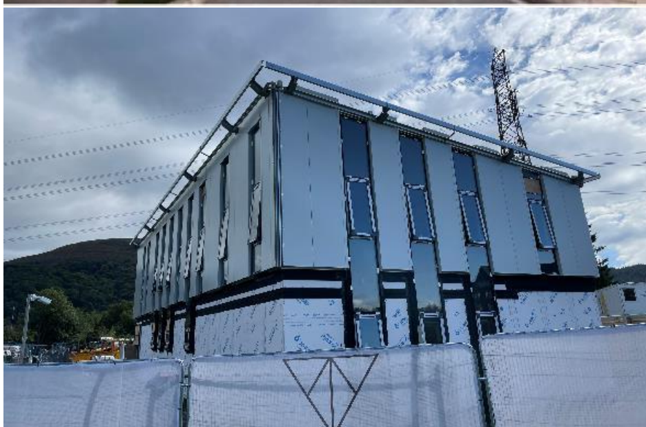
Artist impression of new police station located near A465 at Llanfoist (above) and now under construction (below)
